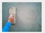
1:4 Ratio Mixture (40kg Bag) Coverage - 16 sq.ft to 20 sq.ft Thickness - 10 mm to 12 mm
